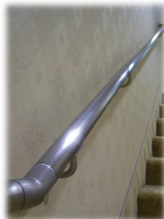
B220 (Round Saddle Included) Fits 1.33" – 1.67" dia Removable Saddle
